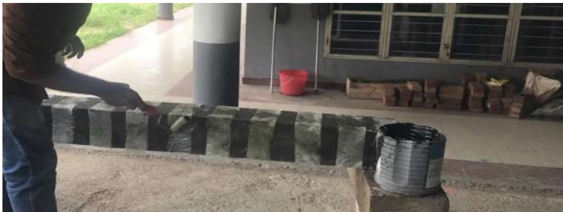
Fig 3.1: Application and fixing of glass fibre sheet and resin mortar
